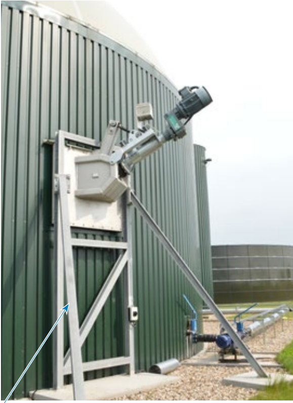
Lower stand member wall construction for use in a steel tank. A consultation is first required to clarify technical details.
